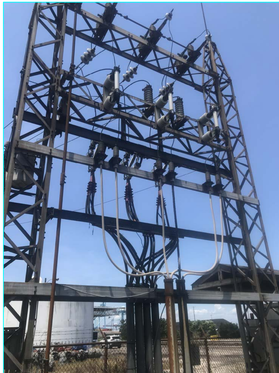
SOUTH SIDE DEAD-END STRUCTURE
