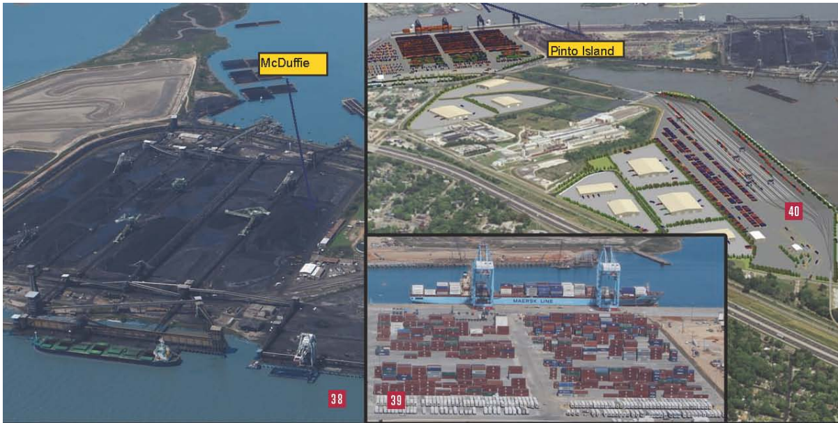
38. McDuffie Terminal; 3065-ft. of berth (three berths); dredged to 45 feet 39. Mobile Container Terminal; 2000-ft. of berth at 45-ft. depth 40. Choctaw Point Complex; intermodal rail and Logistics Park; on-terminal road connection to Mobile Container Terminal; access to 5 Class I railroads
