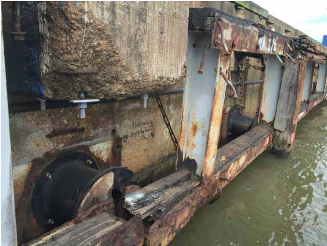
Typical Berth 2 Fender System – Looking Northwest
