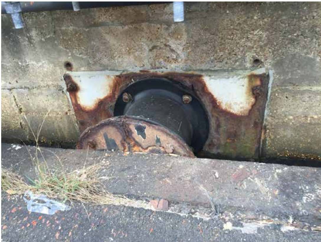
Typical Berth 2 Fender System – Looking West
