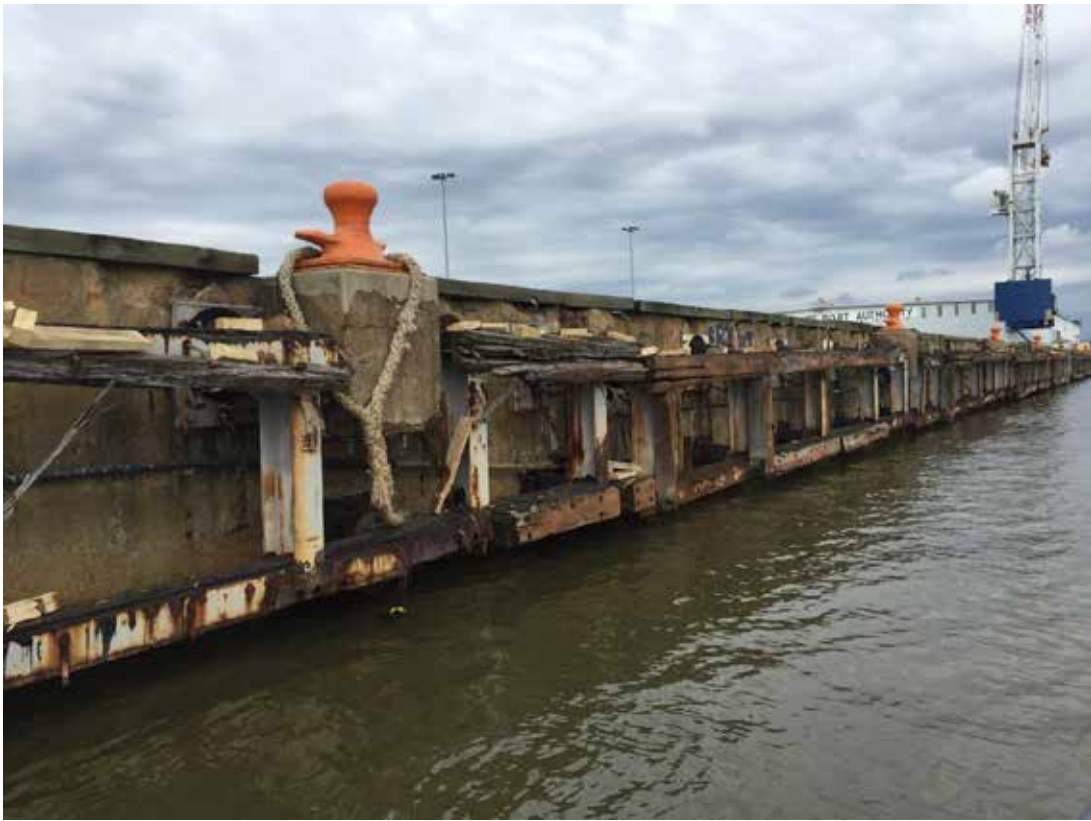
Typical Berth 2 Fender System – Looking Northwest
