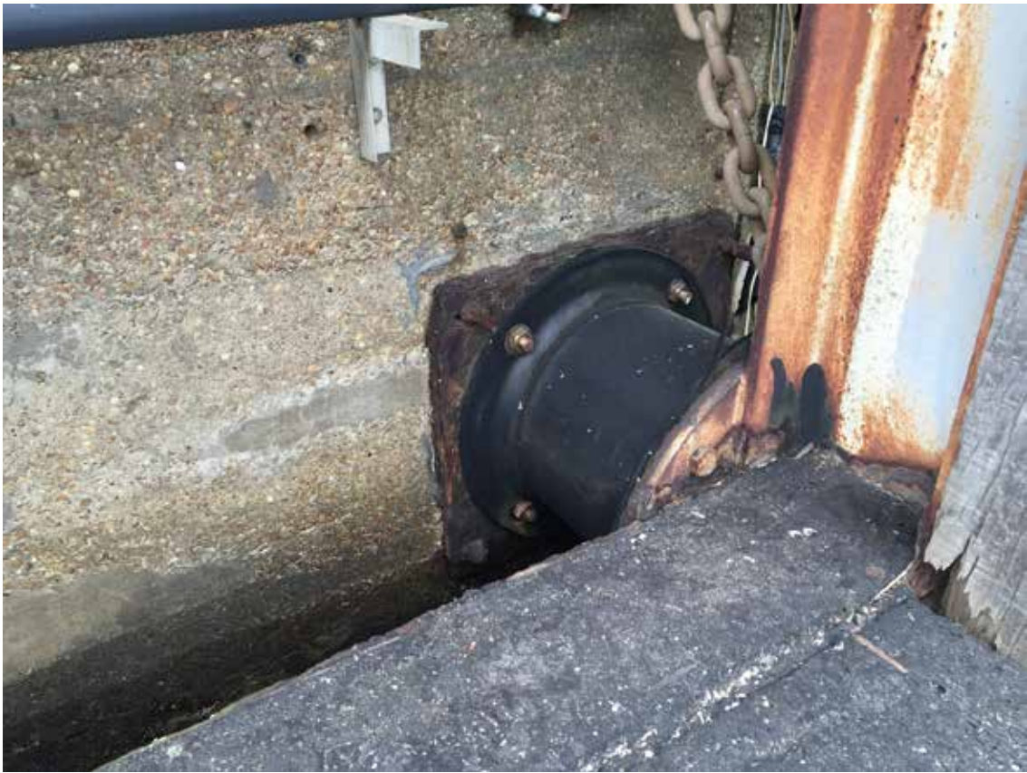
Typical Berth 2 Fender System – Looking West
