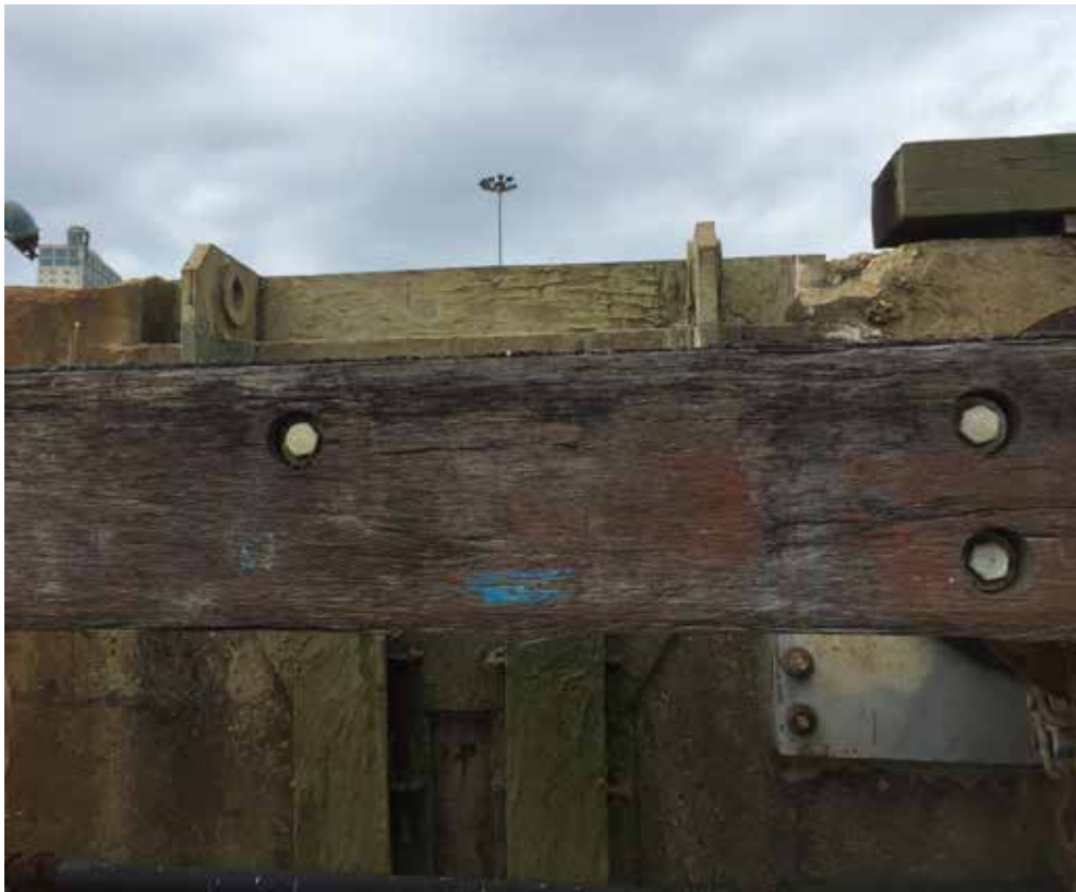
Typical Berth 2 Fender System – Looking West
