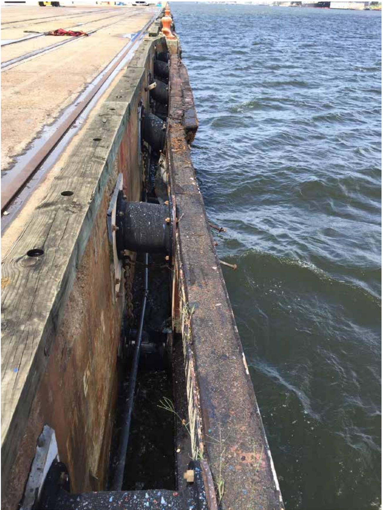
Typical Berth 2 Fender System – Looking North
