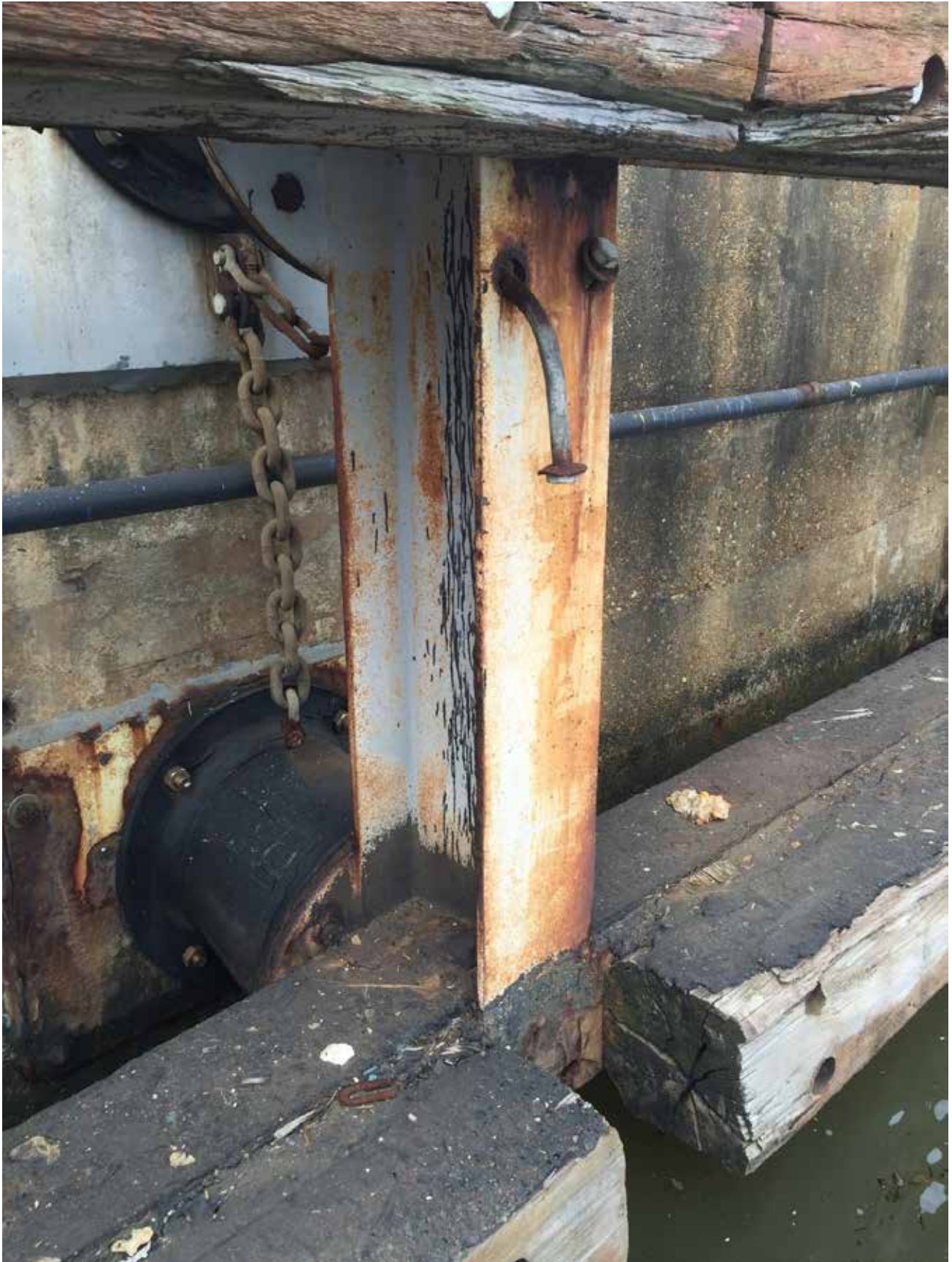
Typical Berth 2 Fender System
