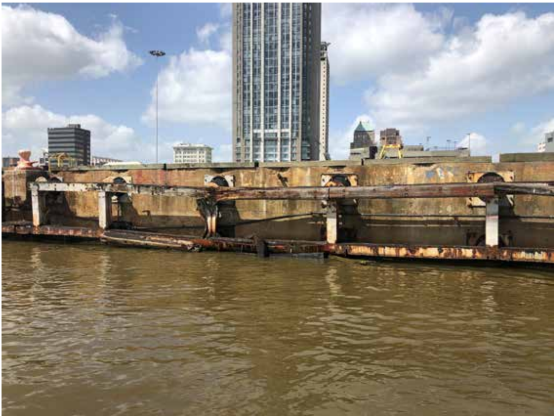
Typical Berth 2 Fender System Between Bollards #6 & #7 – Looking West
