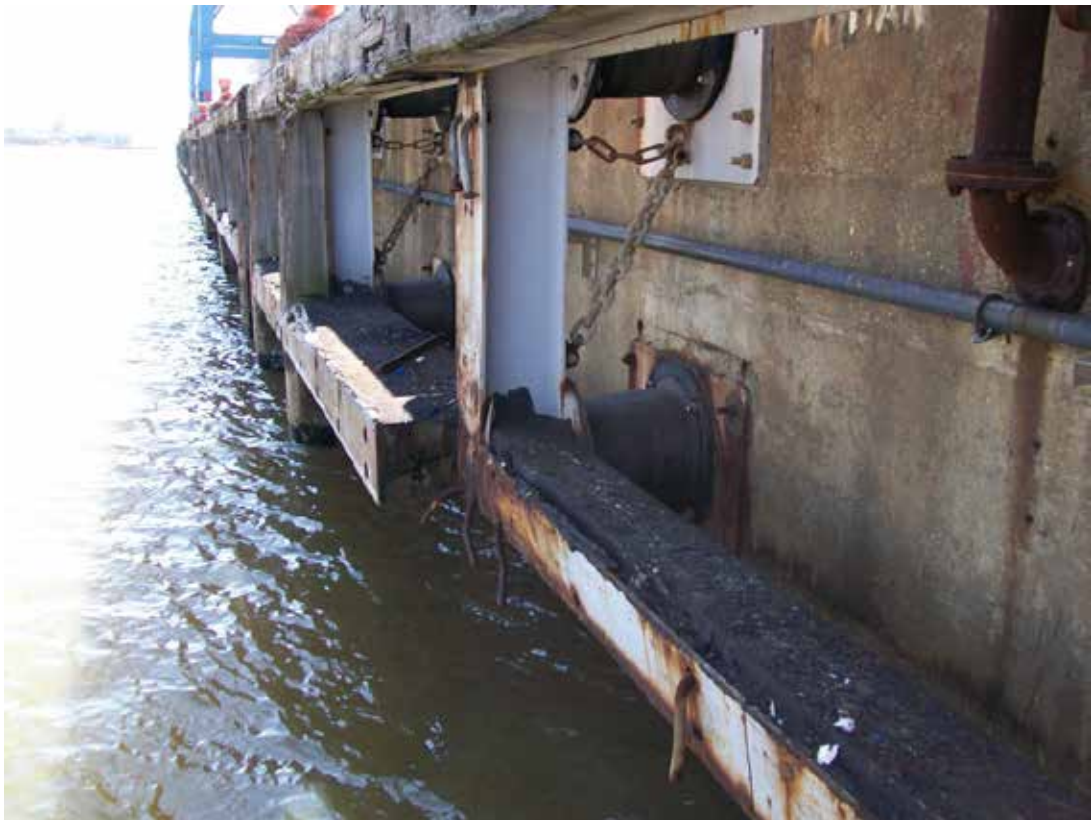
Typical Berth 2 Fender System – Looking South
