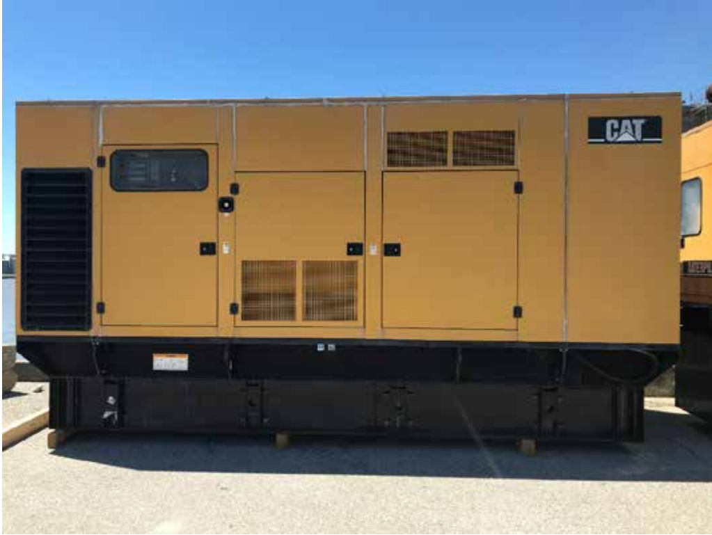
Paceco Crane #246 Generator – Engine Model: 3412 – Serial #: 3FZ08761
