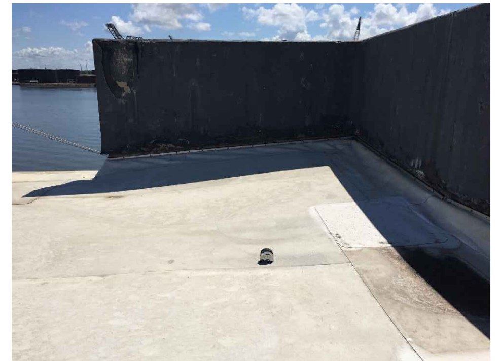
EXISTING CORNER CRICKET AND CONCRETE WALL PHOTO
