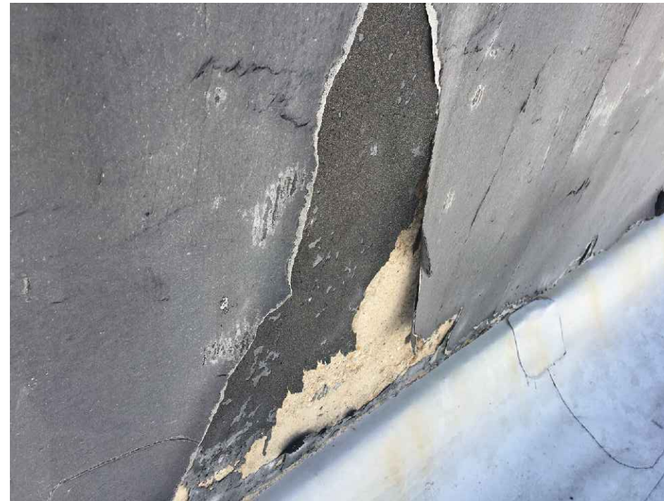
EXISTING CONCRETE WALL SEALANT PHOTO
