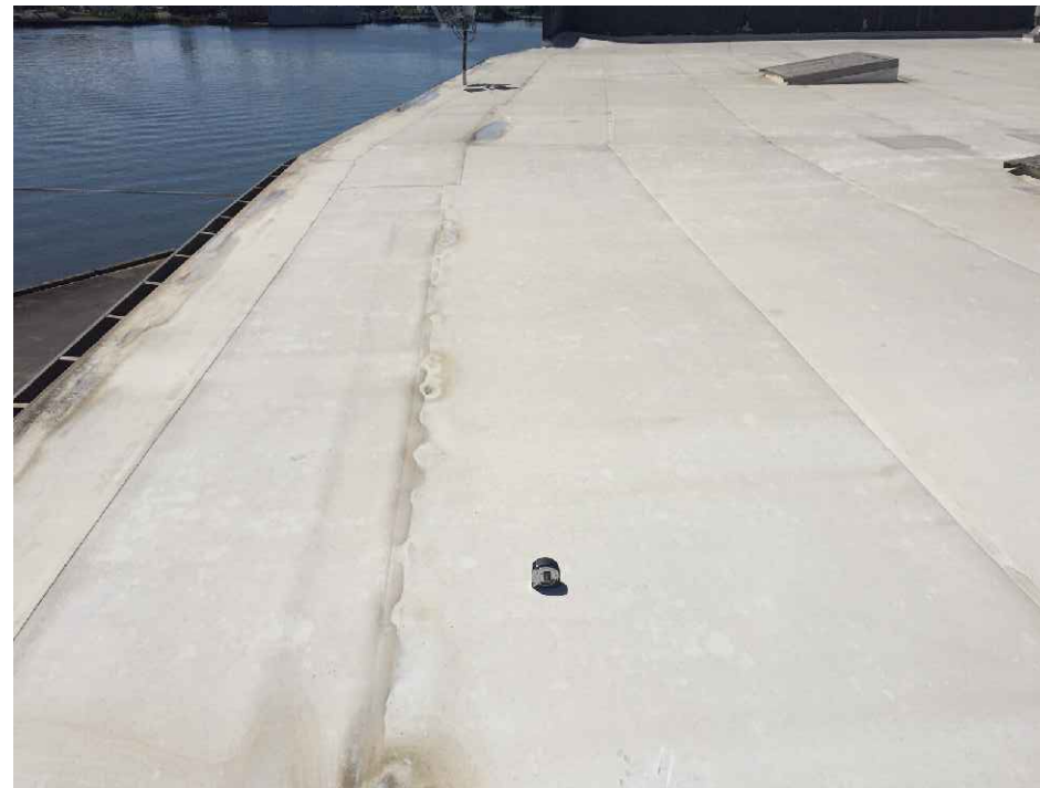
EXISTING ROOF PHOTO
