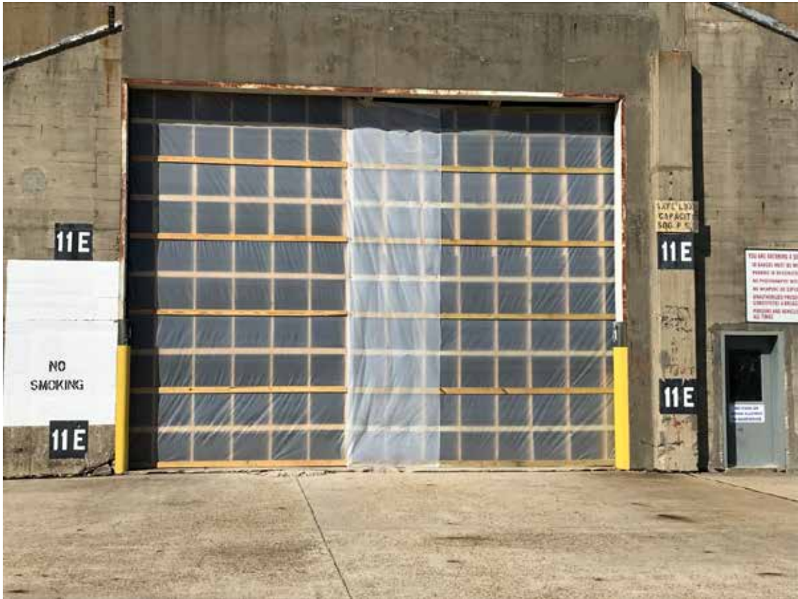
Temporary Door Repairs @ South B-Door 11E
