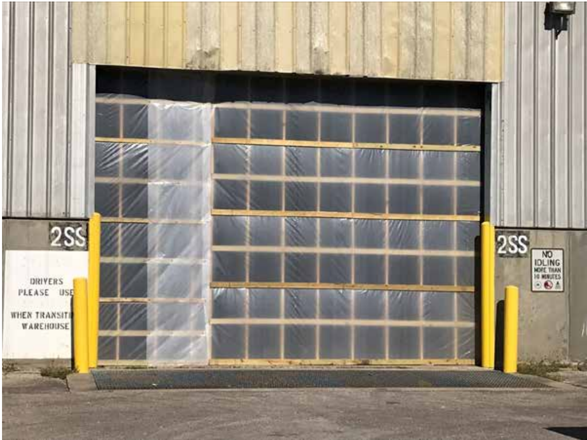
Temporary Door Repairs @ South E-Door 2SS
