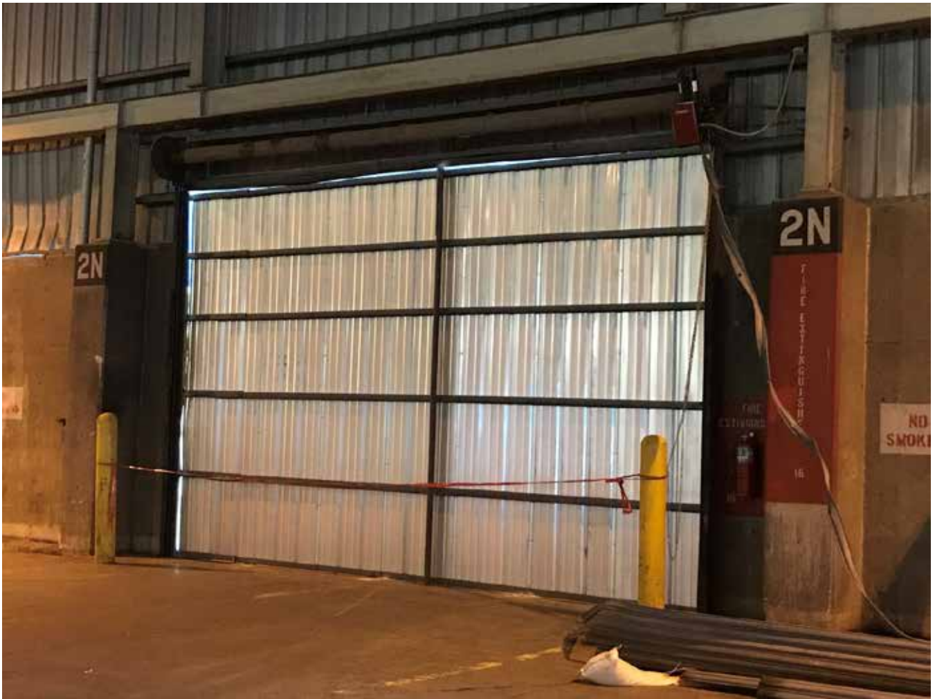
Typical Temporary Repairs North C-Door 2N and North C-Door 4N
