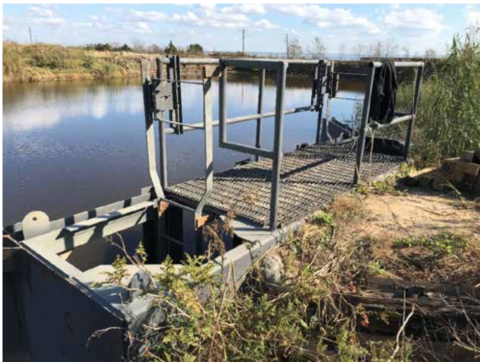
Top of Existing Weir Box
